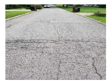
**PCI Range 60-69:** Streets in this category are showing widespread longitudinal, transverse, and alligator cracking. Subgrade distress is evident for the street in areas where the pavement has settled. The surface looks heavily weathered. Characterized by orange in the attached summary.
