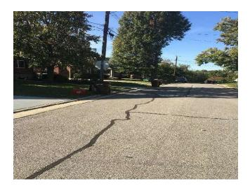
**PCI Range 80-89:** Streets that fall into this category have typically had work performed in the past decade. The asphalt surface has been bleached by the sun and is showing signs of minor cracking. Characterized by green in the attached summary.
