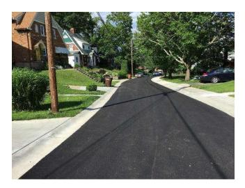
**PCI Range 90-99:** Streets that fall into this category have been recently reconstructed or repaved. The asphalt surface typically appears to be clean, black, and generally devoid of significant defects. Characterized by blue in the attached summary.
