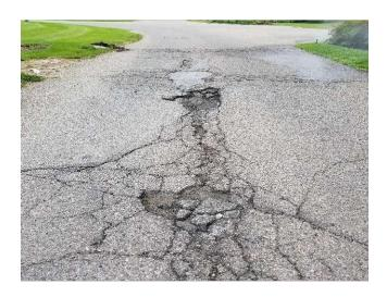
**PCI Range 0-59:** Streets in this category are showing widespread longitudinal, transverse, and alligator cracking. Areas where the pavement has failed are evident from visual inspection. Spots of pavement may be missing. Characterized by red in the attached summary.
