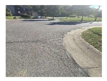
**PCI Range 70-79:** Streets in this category are showing distress in the form of longitudinal, transverse, and alligator cracking. The surface aggregate has started to pop out of the surface and collect at street low points. The surface has a weathered appearance. Some areas may be showing signs of subgrade distress. Characterized by yellow in the attached summary.
